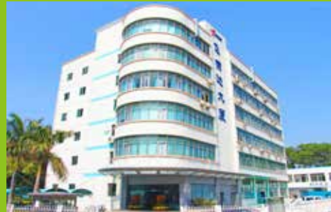
FRD Building (Shenzhen)
