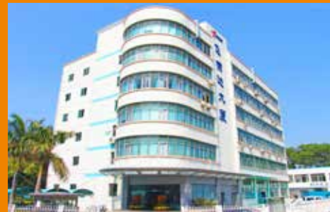
FRD Building (Shenzhen)
